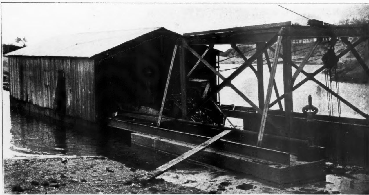
Close Up View of the Dredge. Note the Nozzle in the Right Front. The Hoist is in the Background
